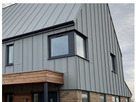
Standing seam zinc
